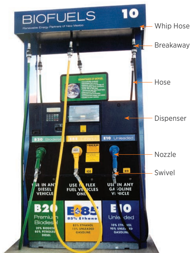
Figure 14. Dispenser and Hanging Hardware.
